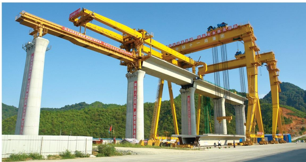
中铁十一局集团锡乌铁路铺架三标项目部 china railway 11 th bureau group Wulanhote-Xilinhot railway track laying project
